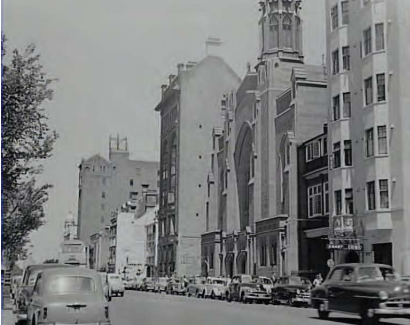
Figure 2.16 View of the western side of Macquarie Street looking south. The facade of St Stephen's Uniting Church is visible in the centre of the image.
