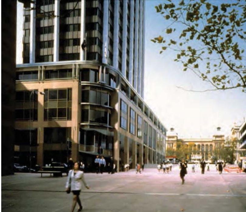
Figure 2.46 A photomontage of the south western corner of the podium prior to its construction in 1998. This image illustrates the relationship with the Sydney Hospital on the eastern side of Macquarie Street, in the background. Martin Place had been closed to vehicular traffic by this stage.
