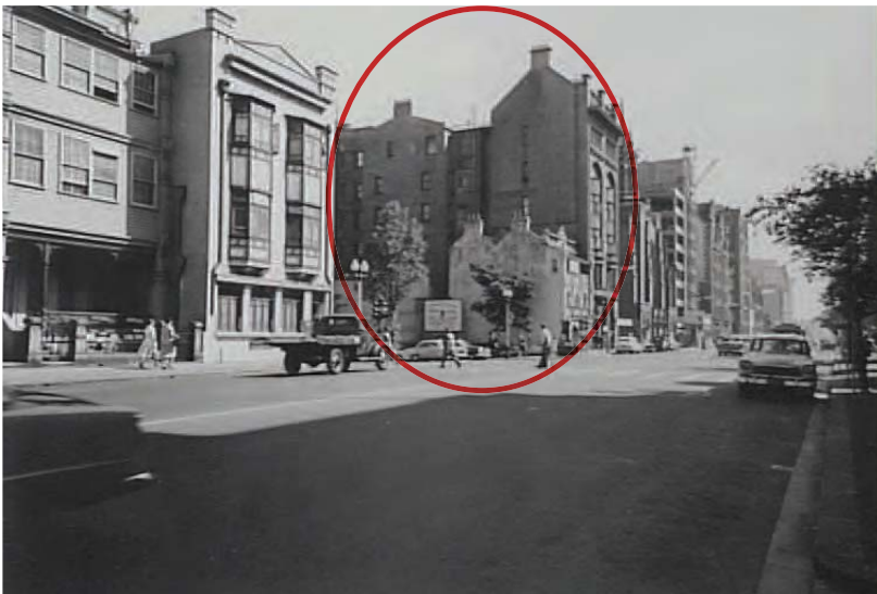
Figure 2.17 View looking north east along Macquarie Street with the Albany (201 Macquarie Street) and St Stephen's Uniting Church to the right of the image. The buildings circled in red in the centre of the image are located on the subject site.
