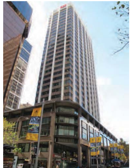
Figure 3.37 The south western corner of the building, as viewed from west of the intersection with Phillip Street, in Martin Place.
