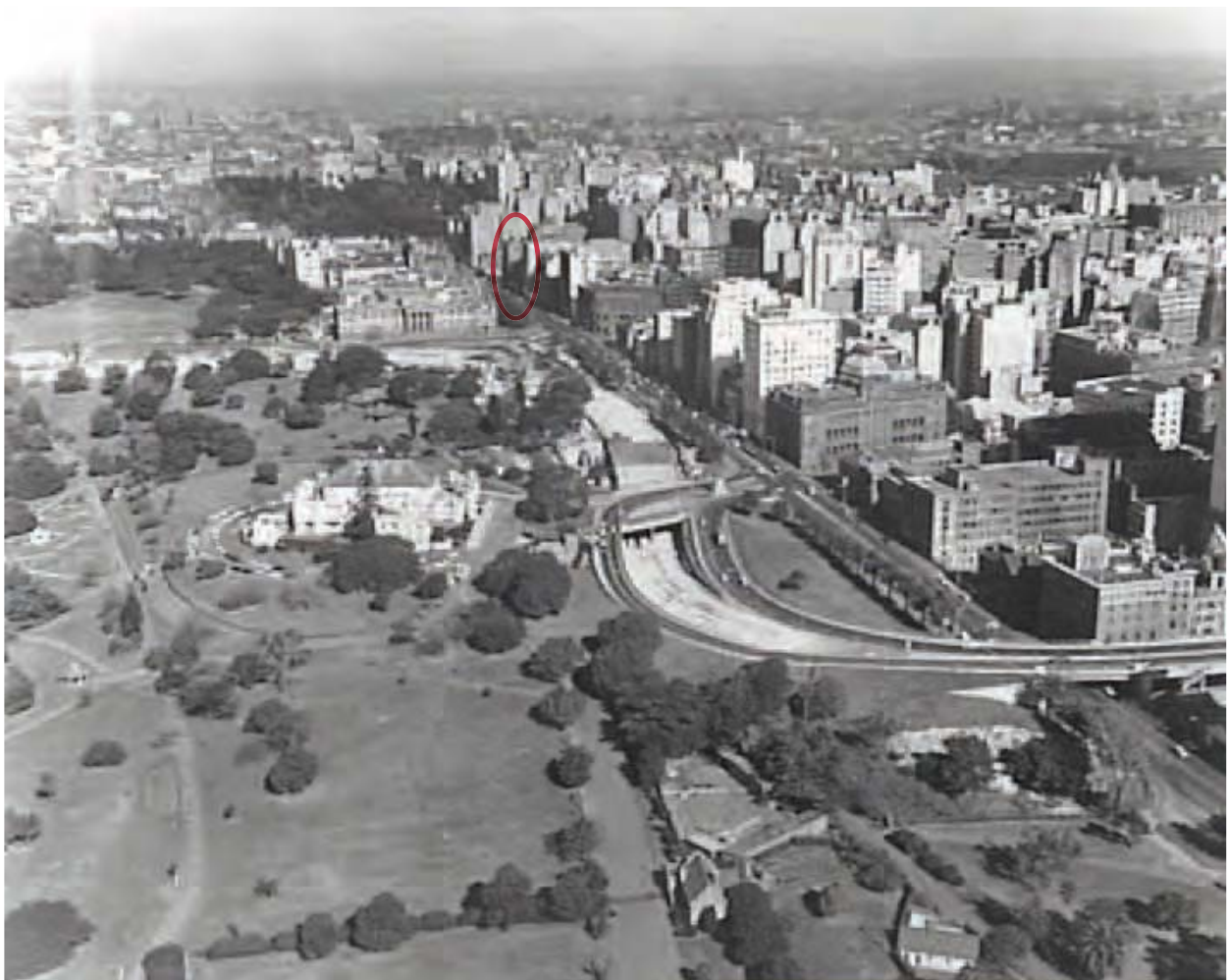
Figure 2.19 An aerial of the Macquarie Street wall, circa 1961. The former 6 storey building on the subject site is circled in red.
