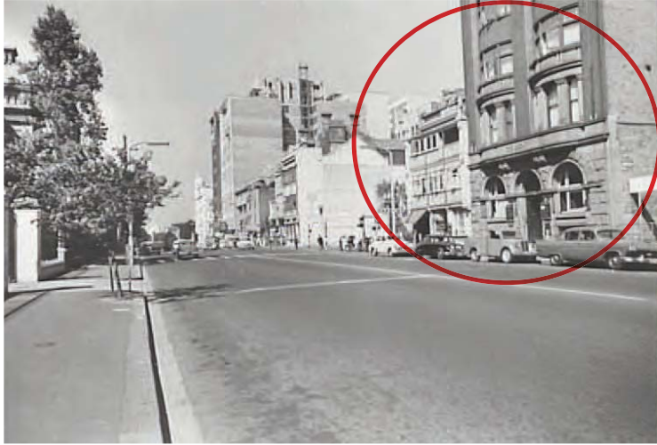
Figure 2.18 View looking south along Macquarie Street, with the Albany (201 Macquarie Street) in the foreground and the Barristers Chambers in the background (239 - 241 Macquarie Street) at the corner of King Street. The three storey terrace and the six storey building, circled red, in the foreground are located on the subject site.
