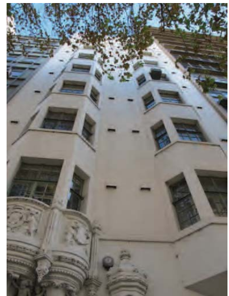
Figure 8.3 Heritage Item, "Hengrove Hall", located at 193 Macquarie Street, Sydney, which is located to the north of the subject site on Macquarie Street.
